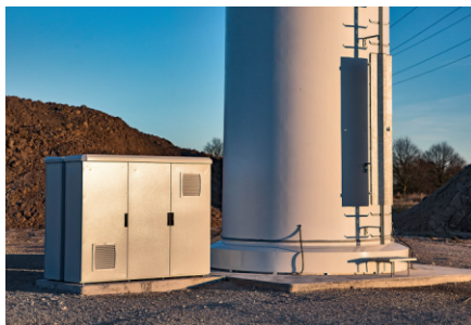
Base for concrete structure
